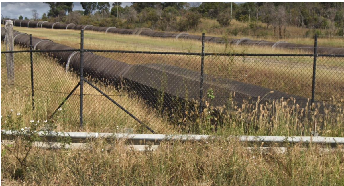
Figure H.1 – Warragamba Pipeline east of Luddenham Road
