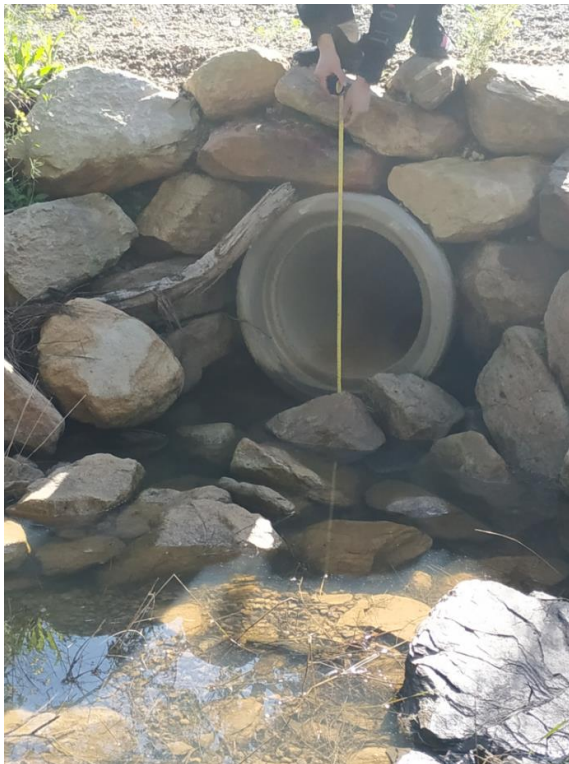
Photo 1 – 0.525m RCP – Paton Lane
